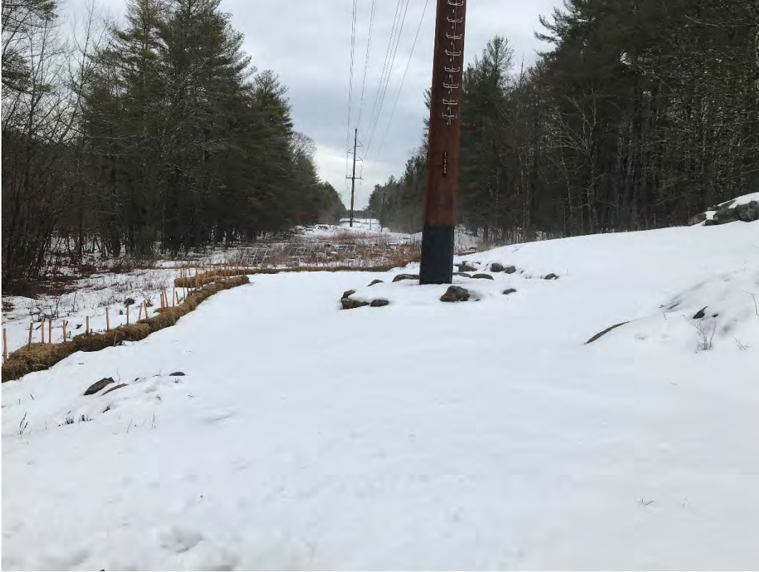
Fig 5: Str. 89 work area. Viewing southeast. (03-01-21)
