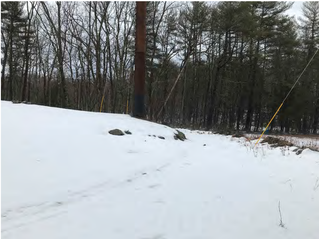
Fig 6: Str. 90 work area. Viewing northeast. (03-01-21)
